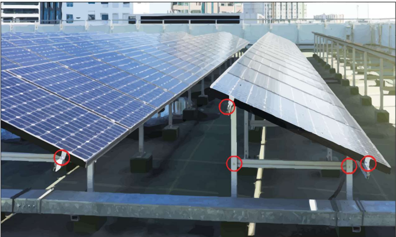
Image 1: The typical PV racking system contains many fastened joints and their performance has a direct impact on the reliability of the overall PV system.
